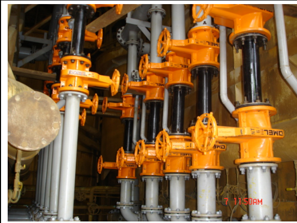
Cavitation Tube installation in 250 m 3 Phosphate Column
