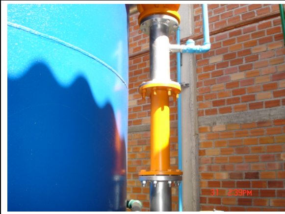
Cavitation Tube installation in 26 m 3 Feldspar Column
