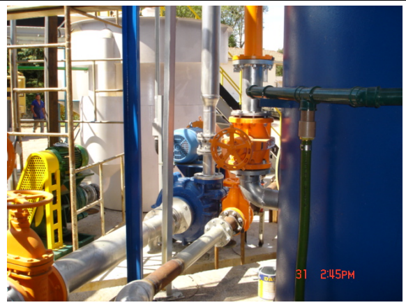
Cavitation Tube installation in 26 m 3 Feldspar Column
