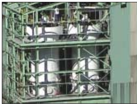
Figure 1. 3m CoalPro columns treating nominal 100x325 mesh feed.
